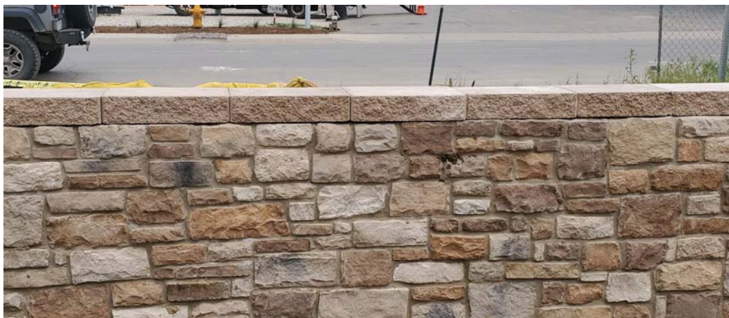
Top of Spillway
