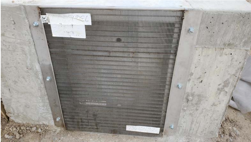
Front of Outlet structure
