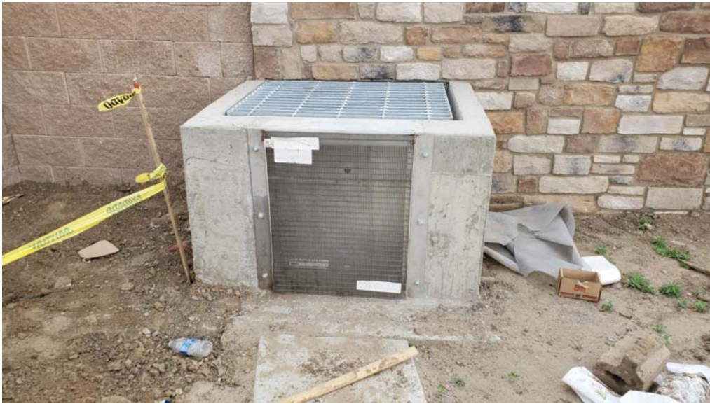
Outlet structure with concrete trickle channel
